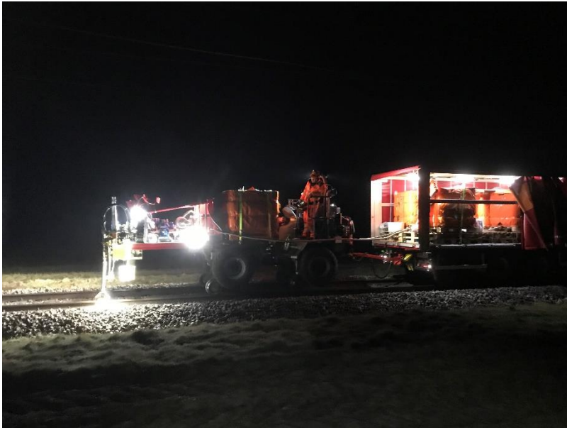
View of the application execution
