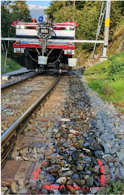
View of ballast bonding on site
