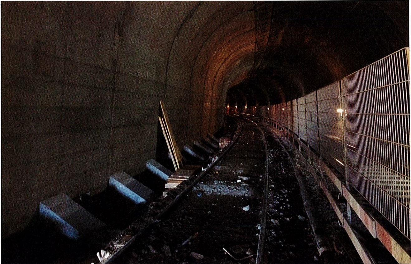
9 Neu angeschlossene Sohlsprenger Newly attached invert spreaders
